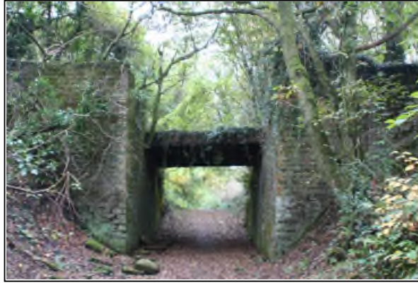
Figure 9 -The Grade II Listed Structures and Bridge
